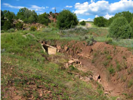
Poorly designed culverts and road drainage systems contribute to erosion and ecological degradation throughout the Basin.
