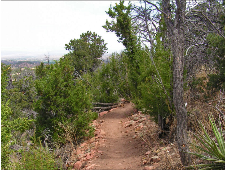
Figure 4. Vegetation restricts sight lines along this trail. Vegetation removal can create adequate visibility, remove dead wood, and open a trail corridor with adequate width. (Photo: Cynthia Lovely)
