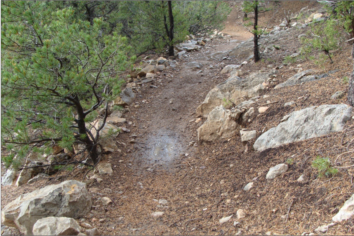
Figure 7. Trails that are not outsloped in drainage areas will allow water to accumulate. Outsloping and removing berms will minimize puddles. (Photo: Cynthia Lovely)
