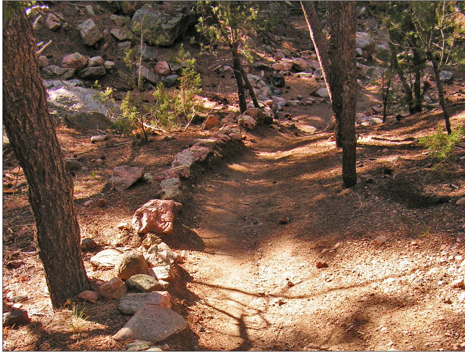
Figure 6. A berm of dirt or rock prevents water from running off the trail. Instead, water will run down the trail, eroding the tread and creating a U-shaped trail profile that increases tread erosion. (Photo: Cynthia Lovely)
