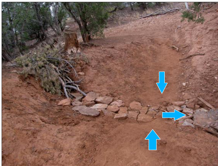
Figure 10. A well placed rolling grade dip (foreground) with a drainage path stabilized by rock. The blue arrows show the direction of water flow. (Photo: Earth Works Institute)
