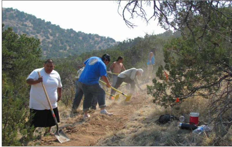
Figure 9. Grubbing a new trail tread for a relocated section of trail. (Photo: Earth Works Institute)
