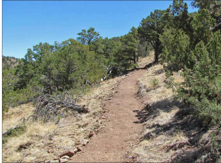
Figure 8. This is an example of a well-brushed trail with good visibility, an interesting “gateway” passage through vegetation, and an outsloped trail tread for optimal drainage. (Photo: Earth Works Institute)
