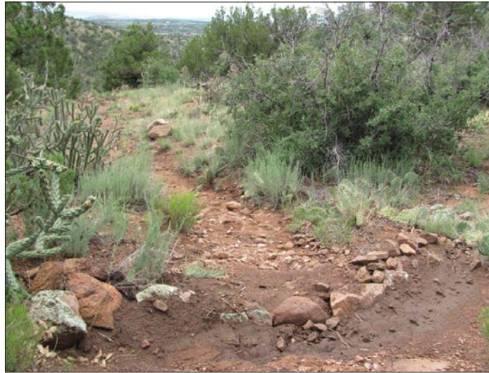
Figure 14. A poorly functioning waterbar with puddling. (Photo: Earth Works Institute)
