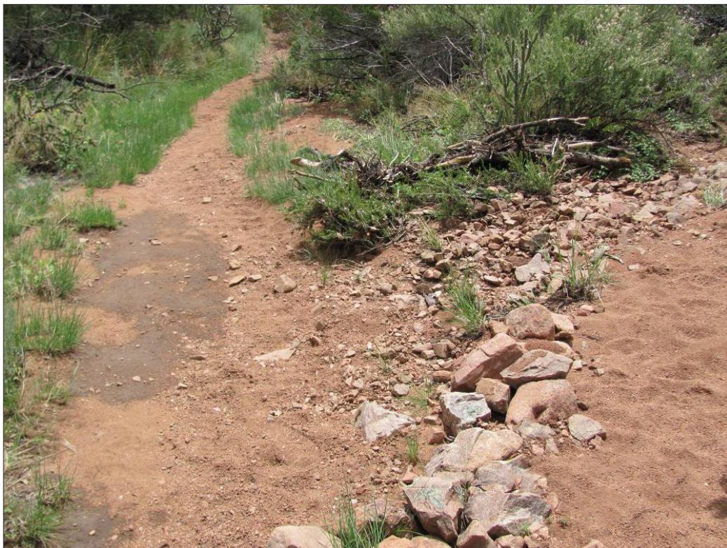
Figure 16. A rock step in a switchback helps scale the steeper grade at this location. (Photo: Earth Works Institute)
