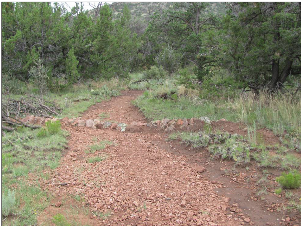
Figure 11. A well-built, effective waterbar. (Photo: Earth Works Institute)
