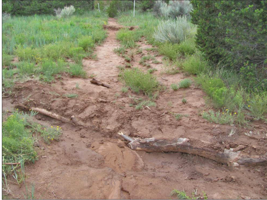
Figure 15. The placement of this waterbar causes trail users to walk around, widening the trail. (Photo: Earth Works Institute)
