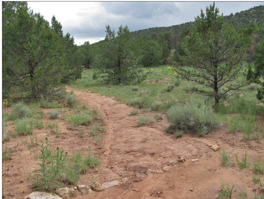
Figure 13. A failing waterbar. (Photo: Earth Works Institute)
