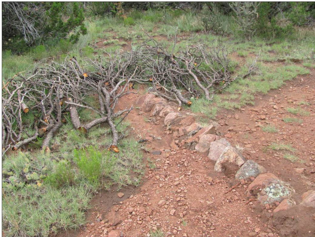
Figure 12. The same waterbar as previous page, showing outflow protection. (Photo: Earth Works Institute)
