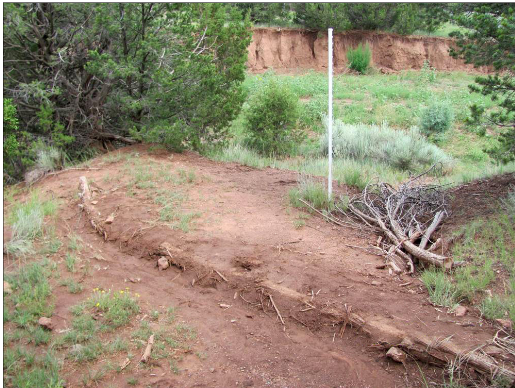
Figure 17. A log waterbar. (Photo: Earth Works Institute)
