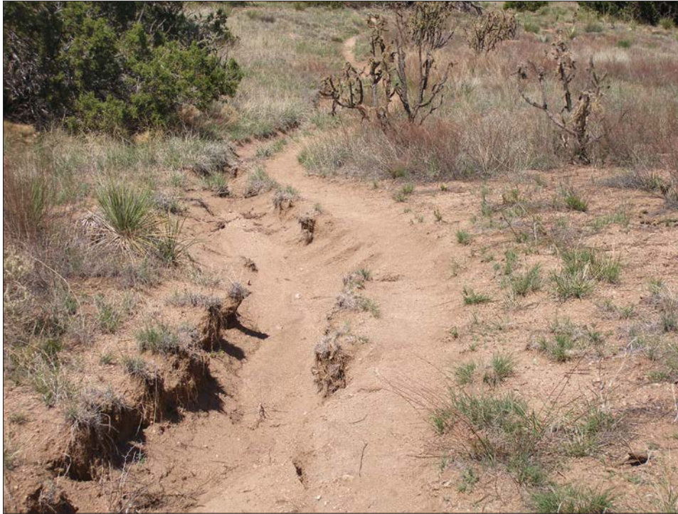
Figure 2. A poorly placed trail located in a natural depression, which has turned the trail into a drainage channel and formed a gully. (Photo: Earth Works Institute)
