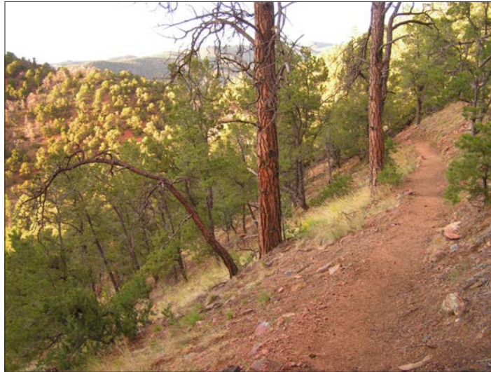
Figure 1. A well-designed and maintained trail, which has a gentle slope and is able to shed water. (Photo: Cynthia Lovely)
